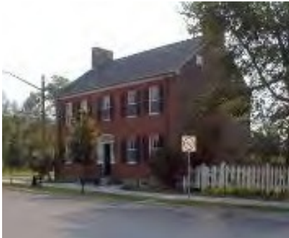
Sheriff Andrews House – contextual view
